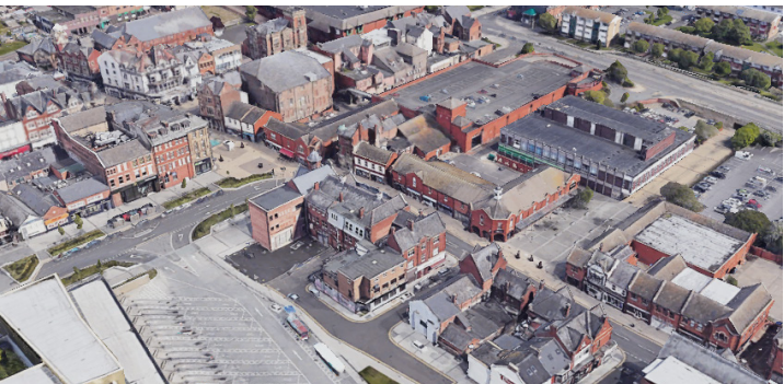
Fig 1.2.3 - Aerial view of site facing north east (site boundary in red)
