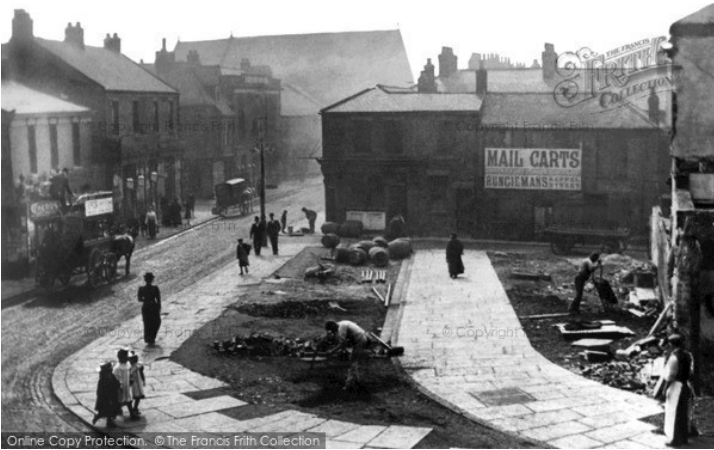
Fig 4 - Photo of Fowler Street facing south. (From early 20th century)
