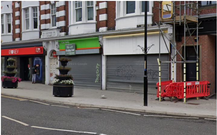
Fig 3.1.1 Vacant commercial units at 24 Fowler Street
