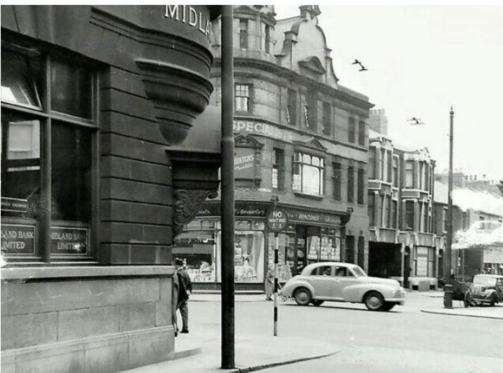
Fig 3 - Photo of 22 Fowler Street from opposite Bank building. (From mid 20th century)
