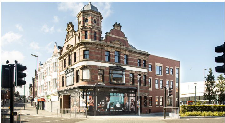
Fig 3.1.3 Recent conversion of 22 Fowler street to refurbish shopfront and provide residential units
