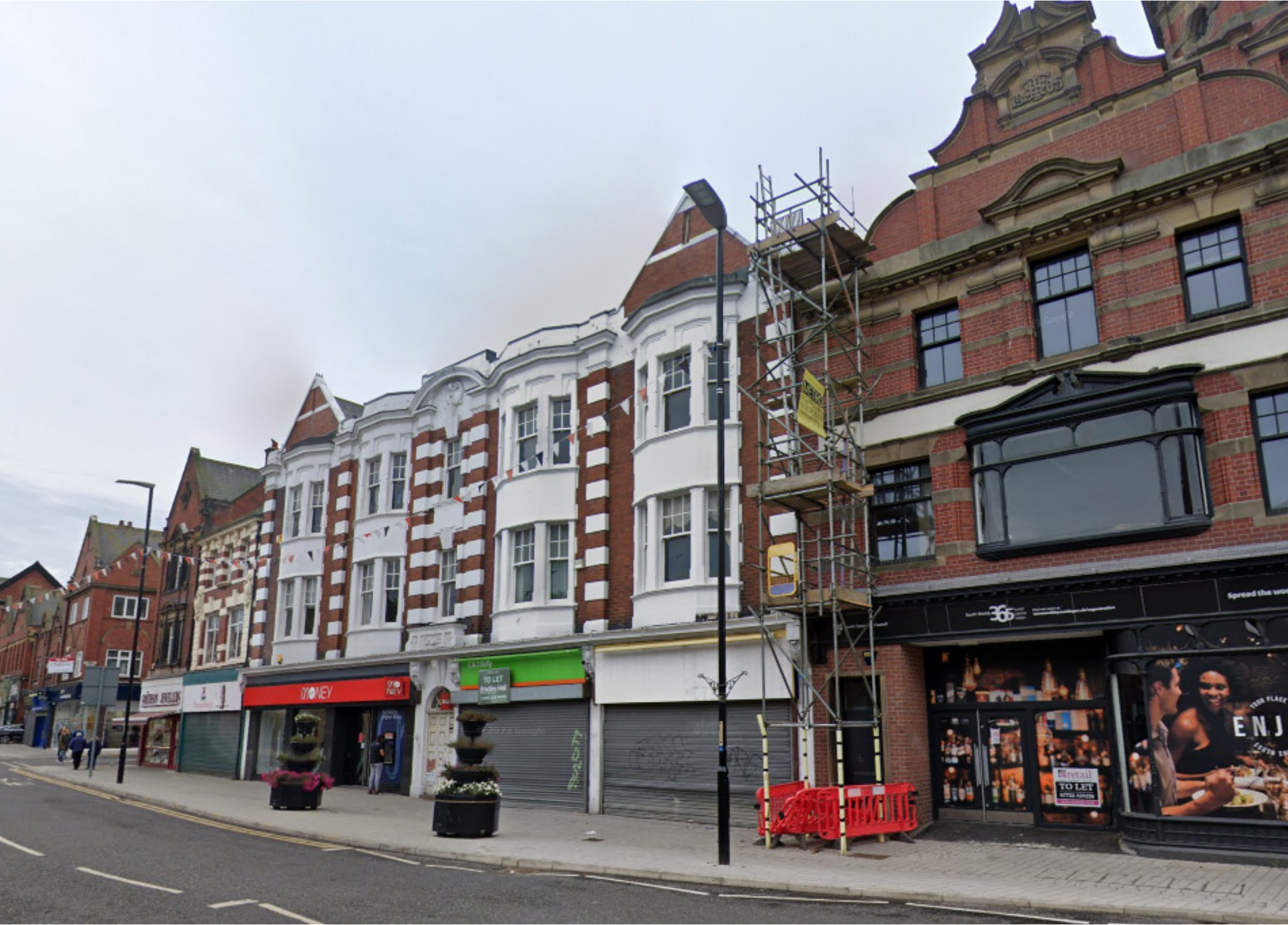
Fig 1.1.1 - Street view of front facade of building
